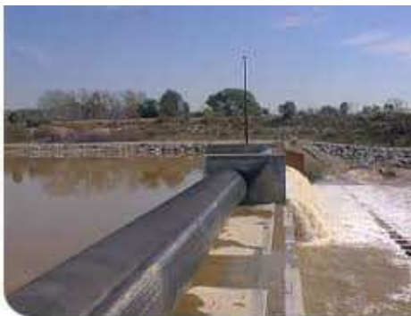
Figure 3.10. Illustration of inflatable (rubber) weir.
