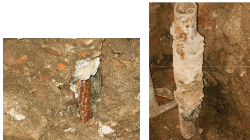
Fig. 2. Dug-up piles reinforced with steel tubes
