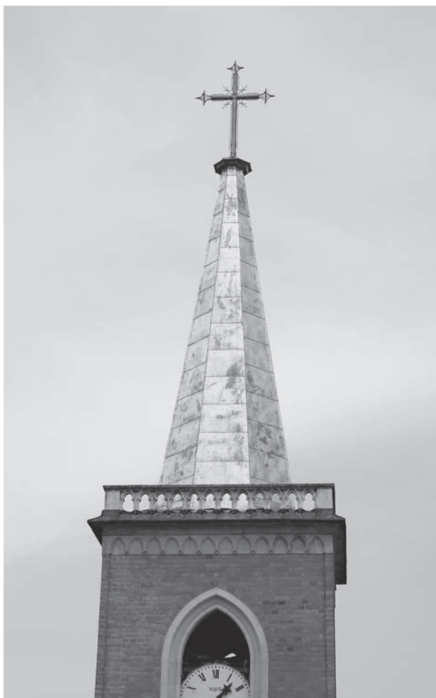
Fig. 5. Final stage of the tower copula renovation surmounted by the cross
