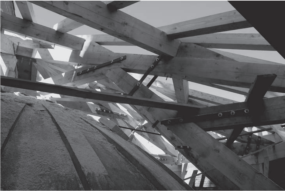
Fig. 4. One of the fixing stages of the roof truss above the presbytery
