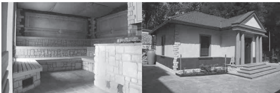
Fig. 5. External sauna for many users at the Saturn's Palace complex in Czeladź (photo by Tomasz Bradecki, 2012)
