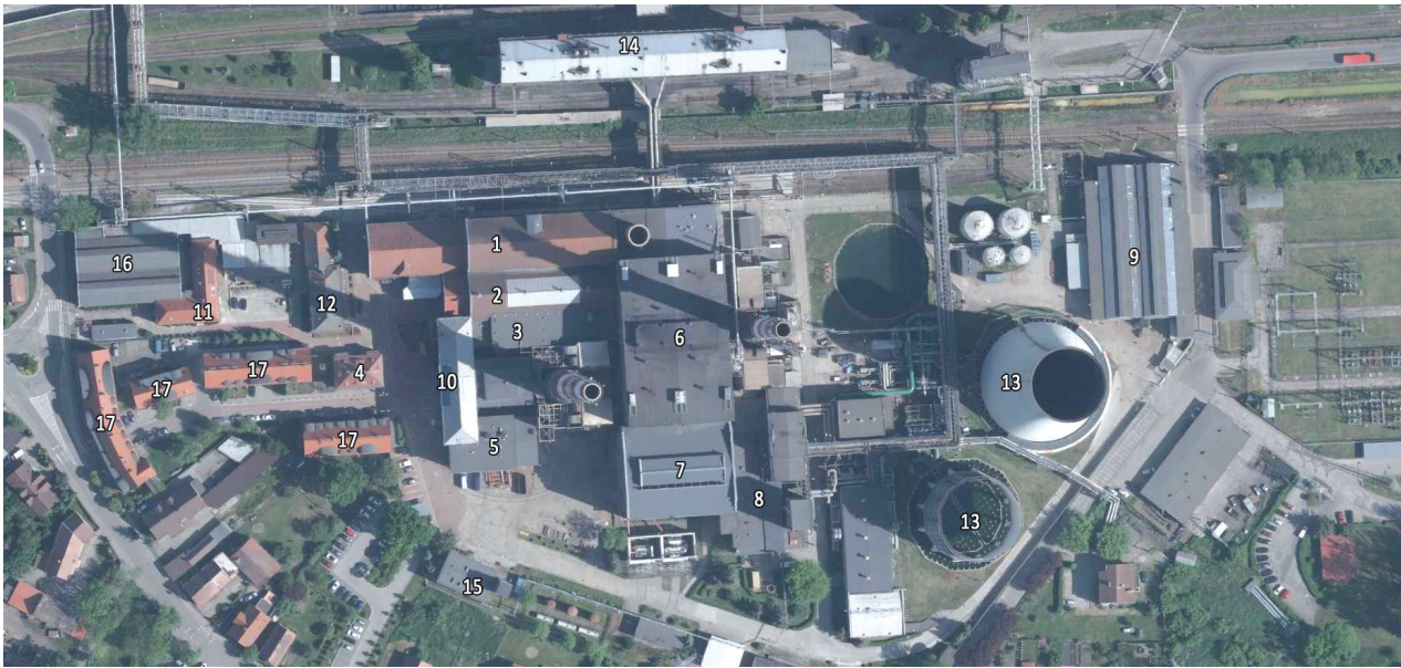
Fig. 2. Top view of the Czechnica CHP Plant, 2018,
