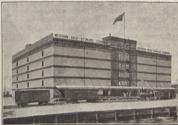
Kaltlagerhaus der Western Cold Storage Company zu Chicago.
