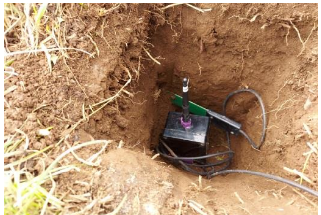
Figure 2. Buried sensor node measuring the moisture of the soil and emitting the data through radio communication
