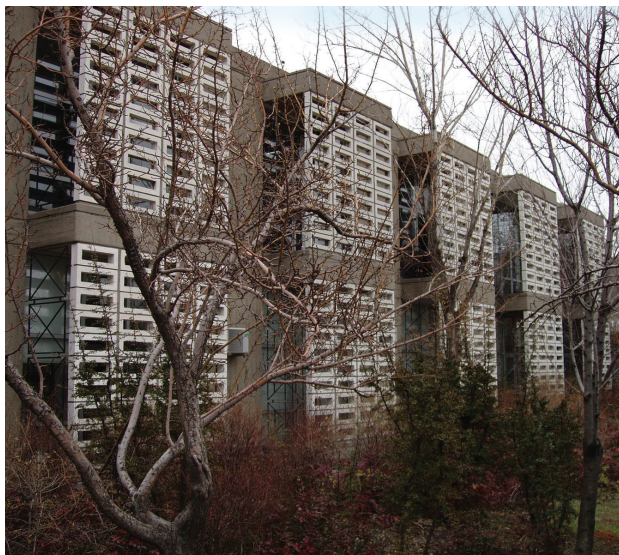
Fig. 8. Altuğ and Behruz Çinici, METU Faculty of Architecture Building in Ankara – sun-breakers in front of the balconies (photo by W. Niebrzydowski)
