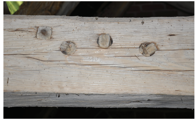
Fig. 5. Kamień Pomorski, cathedral, roof truss over the nave, building material with traces of float in the form of round holes with the remains of wedges and withes (elaborated by U. Schaaf, M. Prarat)
