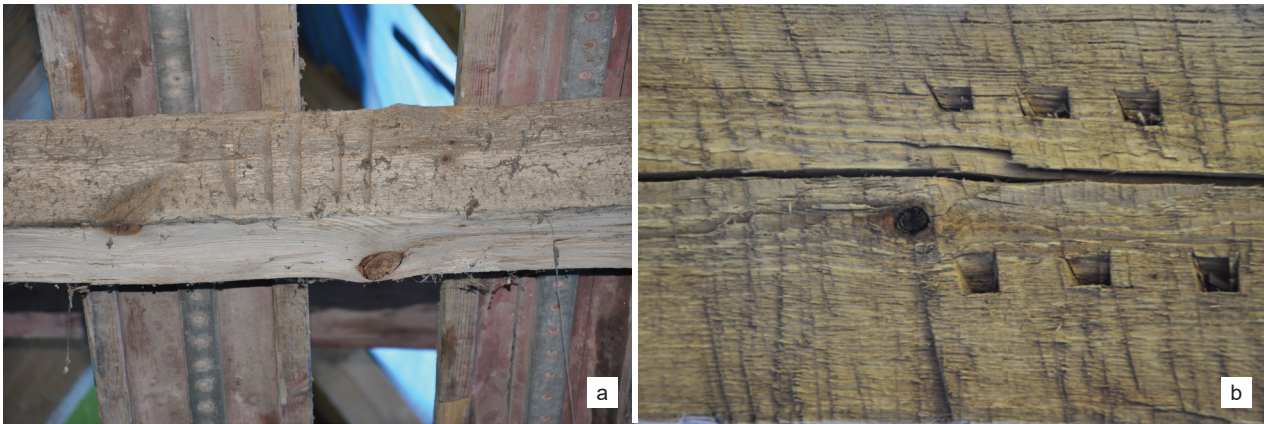
Fig. 3. Kamień Pomorski, cathedral, roof structure above the nave: a) assembly mark in the form of straight lines made with a hand axe, b) assembly mark in the form of rectangular cuts made with a chisel, building material processed from the side of timber framing with a hand saw (photo by U. Schaaf, M. Prarat)
