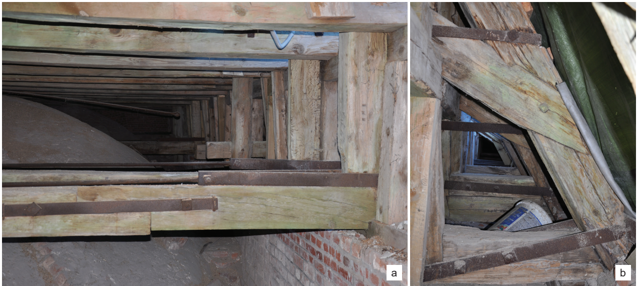
Fig. 9. Kamień Pomorski, cathedral, roof structure above the nave: a) reinforcement of the connection of two parts of the tie beam (principal rafter truss 20) with a flat bar, securing the principal rafter trusses with tensile-resistant anchors (19–20) above the principal rafter truss beam, b) connecting the sole piece with the rafter using two flat bars, joining the (secondary) upper plate with the passing brace and rafter using a flat bar (photo by U. Schaaf, M. Prarat)
