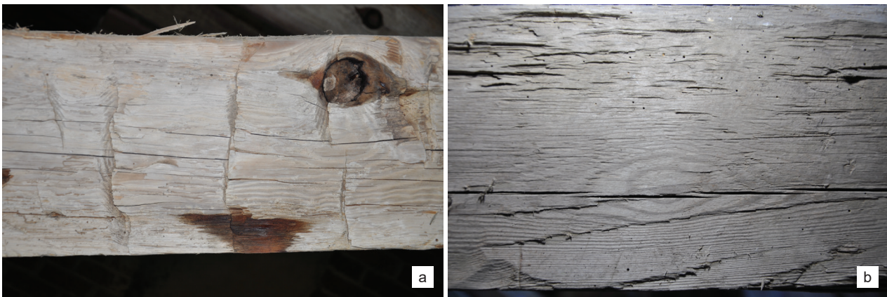
Fig. 4. Kamień Pomorski, cathedral, roof structure above the nave: a) initial processing of wooden building material made with an axe, b) smoothing of pre-processed wooden building material made with an adze (photo by U. Schaaf, M. Prarat)
