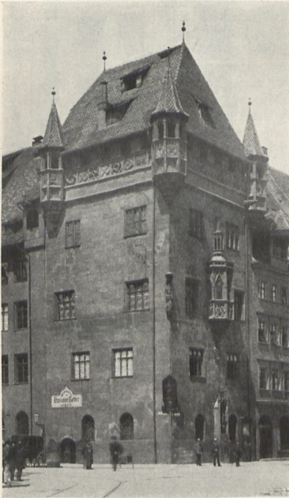
Schlüsselfelder'sches Haus zu Nürnberg.
