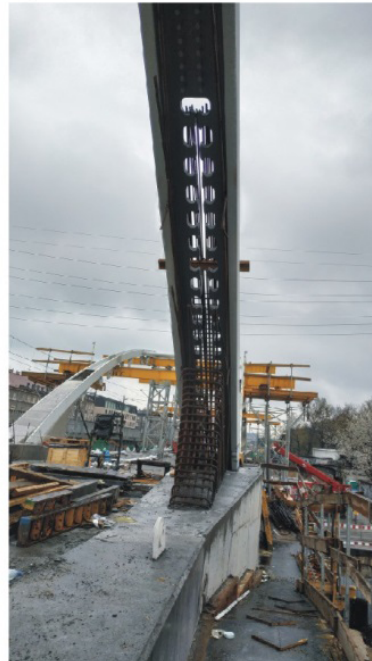
Figure 25: Implementation of composite dowels in innovative composite bridges in Poland: a) and b) implementation in beams – bridge in Elbląg (presented in [41]) and c) implementation in arches – a new solution as part of a network arch bridge using composite dowels [63].
