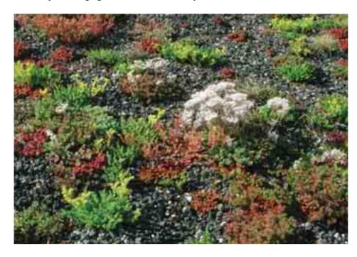
Fig. 1. Sedum cover on extensive roof one year after planting (photo: Mark Depreeuw)
