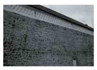
Fig. 9. The west part of the cloister walls from bishop Radziwiłł's time with junction of walls, the so-called toothing, after the preservation in 2008 (photo: O.M. Przybyłowicz)
