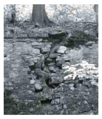
Fig. 17. Destructive influence of plants on the construction structure (photo: J. Potyrała)
