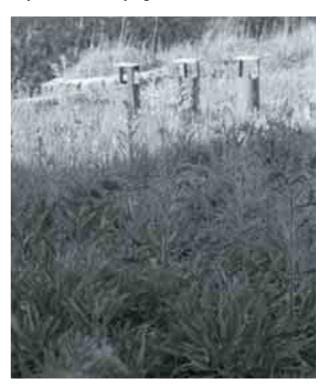
Fig. 2. Various vegetation on a brownroof over staff facilities building in syenite mine in Niemcza, Poland. The picture is taken a year after the soil from the surroundings was elevated onto the roof. No vegetation was planted (photo: M. Baborska-Narożny)
