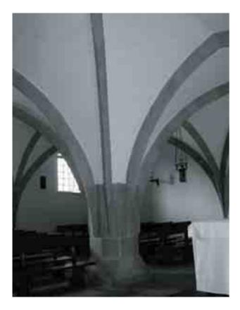
Fig. 3. The old monastic chapter house of 13/14<sup>th</sup> c.with main column, cantilever and leading out of the ribs (photo: O.M. Przybyłowicz)
