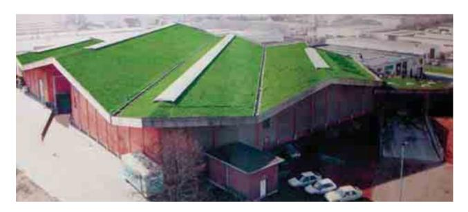
Fig. 6. General view of Ecover factory in Oostmalle. The picture shows grass on the roof which was later exchanged for sedum (photo: archive of Mark Depreeuw)
