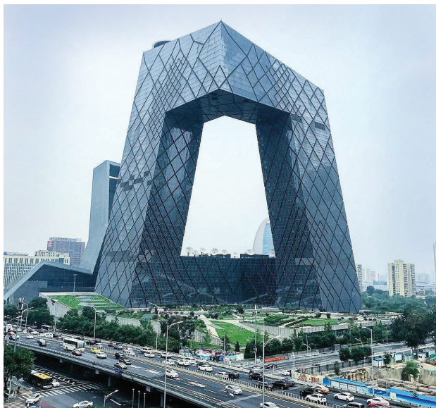
Fig. 1. CCTV building designed by Rem Koolhaas, Beijing, 2012 (photo by Colin Charles, CC BY-NC-ND 2.0, source: flickr.com/photos/byte/35966604971, accessed December 3, 2024)
