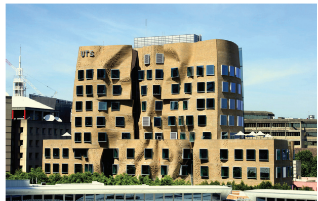
Fig. 4. Dr Chau Chak Wing Building designed by Frank Gehry (Sydney, 2015). Instead of the human side of architecture declared by the author, Simone Brott sees the resemblance to the moment of demolition of the Priut-Igoe (photo by Brickworks Building Products, CC BY-SA 2.0, source: https://tiny.pl/0y5kgd0x , accessed December 3, 2024)
