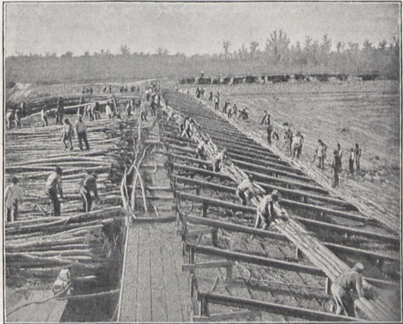
FIG. 2.—Constructing Fascine Mat on Mattress Ways
