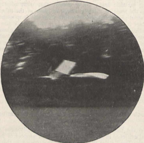
FIG. 2.—Same engine and boiler as before, attached to two inclined wing planes, and tail. From tip to tip of wings 11 feet; total surface of wings and tail about 22 square feet. Total weight of whole apparatus 34 lb. Steam raised to 50 lb. per square inch, and started. Length of flight about 100 yards on level; maximum height during flight, about 20 feet. The propelling screw is seen in front and above the frame.
