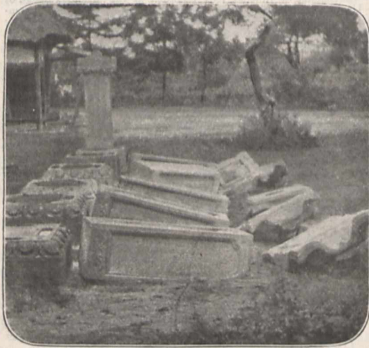
FIG. 4.—Gravestone as seismometers, indicating direction and intensity of movement. (Omori.)
