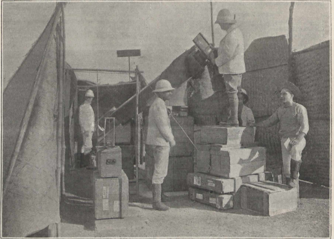
FIG. 3.—9-inch Prismatic Camera, showing arrangement and kind of shelter used.
