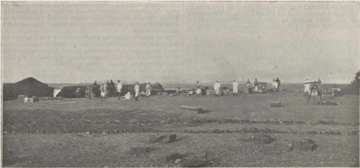
FIG. 1.—Camp, Saturday, January 8. Putting in concrete pillars.
