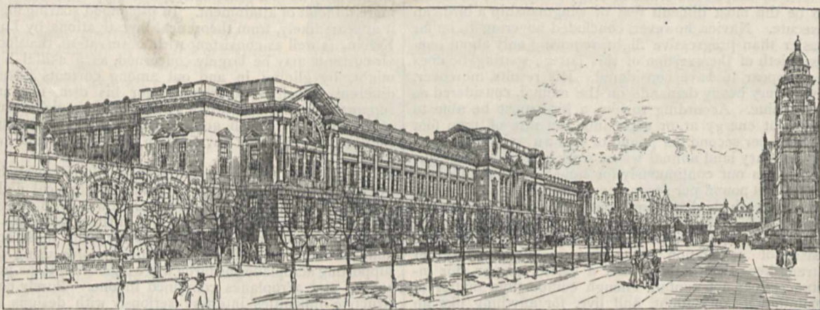
First sketch of proposed Royal College of Science, South Kensington. View from Imperial Institute Road.
