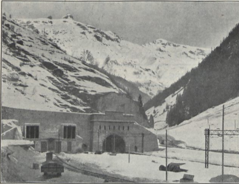
Tunnelportal in Goppenstein.
