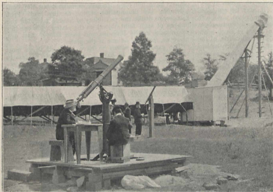
FIG. 1.—Portion of Smithsonian Astrophysical Observatory Eclipse Camp, showing a part of the large 135-foot telescope (under canvas), the 38-foot coronagraph, and the 5-inch equatorial.
