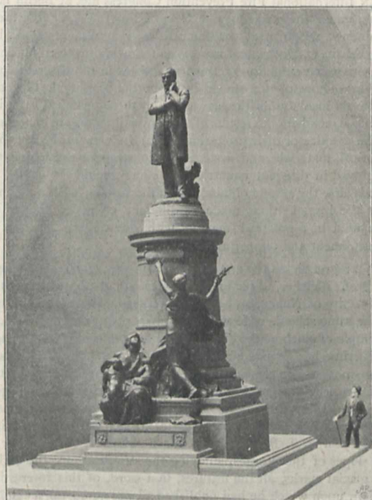
Monument to Pasteur, to be erected at Dôle.
