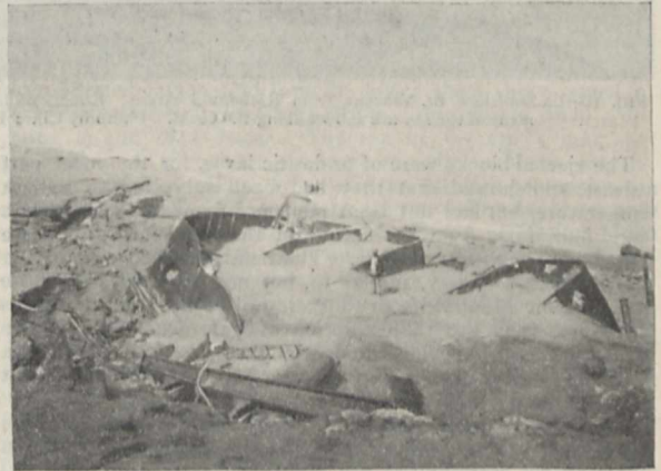
FIG. 3.—Quarter-inch boiler-iron tanks in a distillery in the Fort Quartier of St. Pierre, showing holes made by bombardment of stones from Mont Pelée eruption. Photo by E. O. Hovey.
