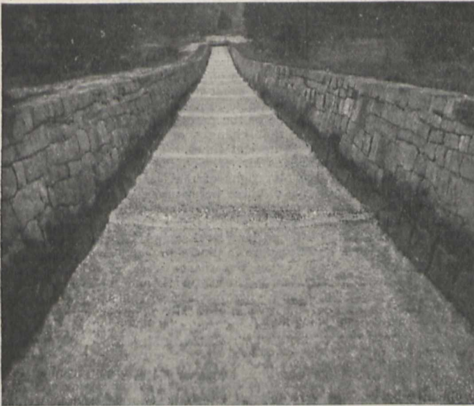
FIG. 1.—A Roll Wave leaping the Outfall of the Grünbach Conduit.
