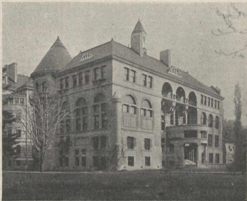
FIG. 1.—Macdonald Physics Building, McGill University, Montreal.
