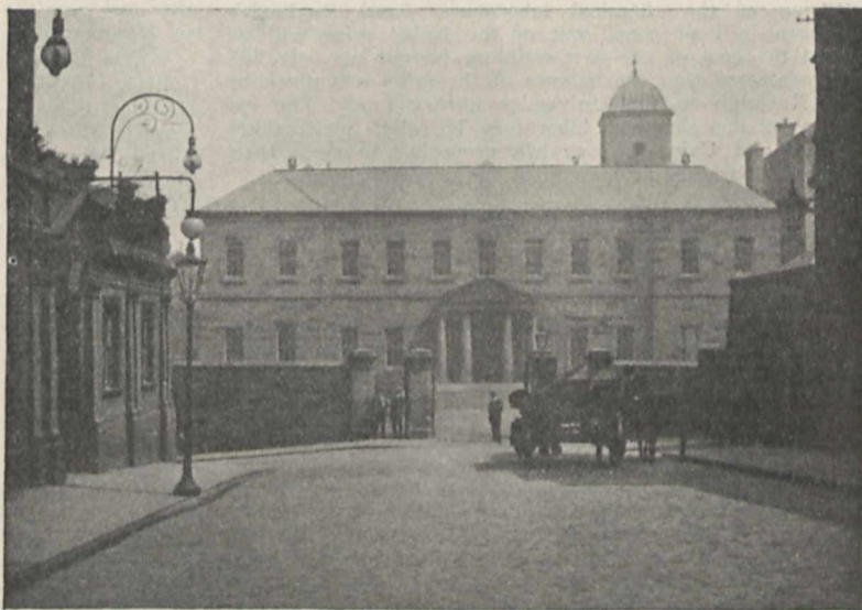
FIG. 2.—Entrance and West Front of new Engineering Department, University of Edinburgh.
