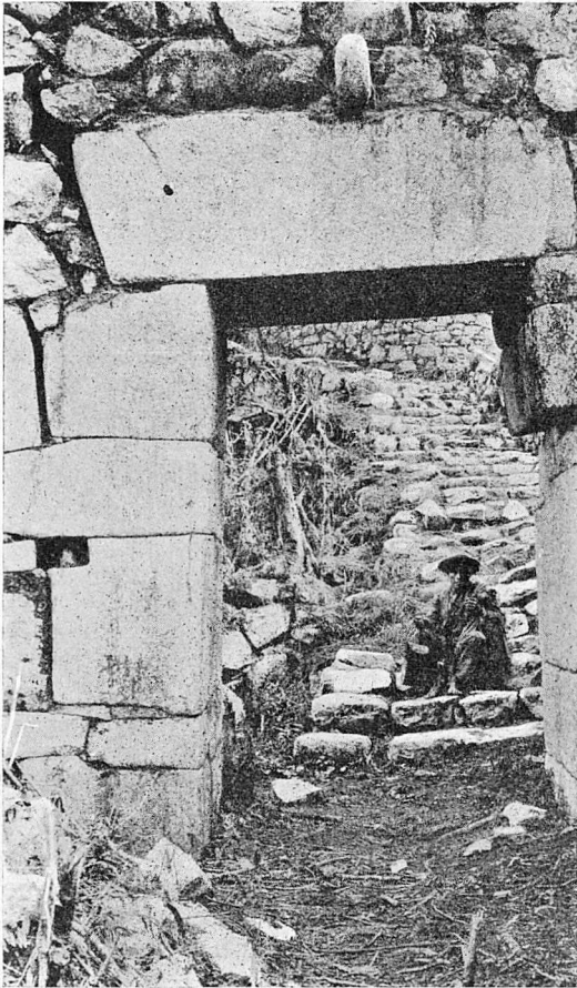
FIG. 5.—Machu Picchu. City gate, interior. Notice the lock hole containing granite cylinder on left and projecting ring stone over the lintel of the doorway. The gate, probably of wood, was either swung from the ring stone or fastened to it and balanced by a log fastened to the stone cylinders in the lock hole on either side of the gateway. A similar device was used also in the entrance doors to each isolated group of houses. Copyright by the National Geographic Society.
