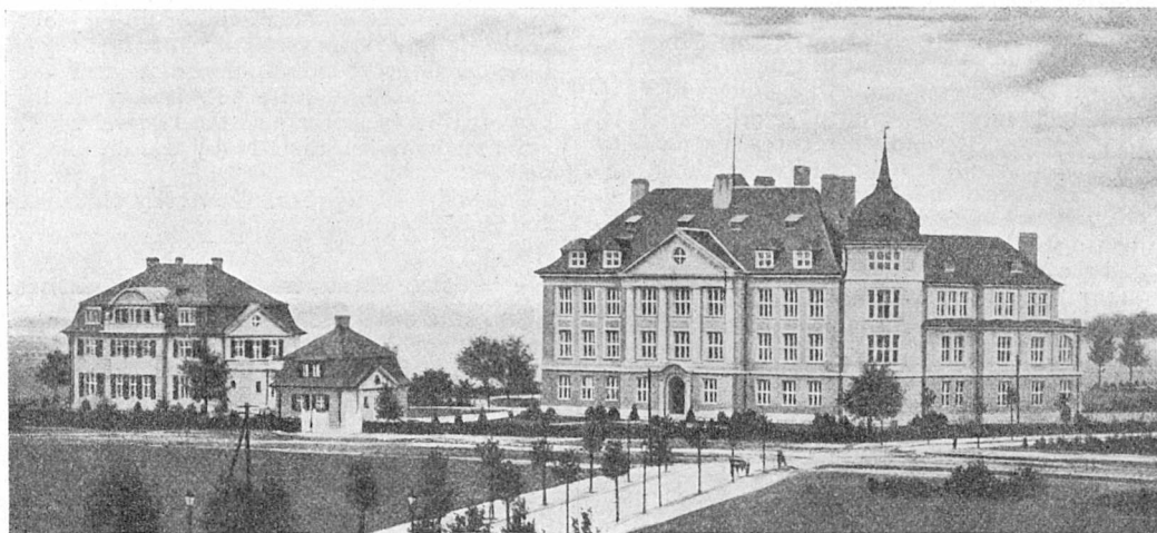
Main building, with director's and porter's houses, of the Kaiser-Wilhelm Institut, Berlin, Dahlem.
