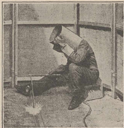
FIG. 2.—Repairing a tram-rail by arc welding, using an iron electrode.
