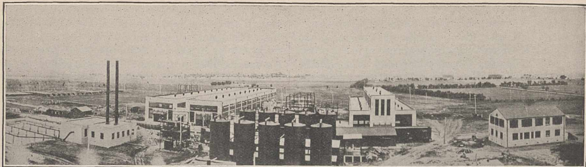
FIG. 1.—Helium production plant, Fort Worth, Texas, operating at the present time.
