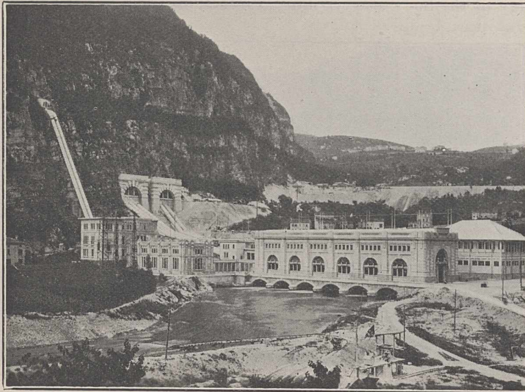
FIG. 2.—Hydro-electric station at Fadalto.
