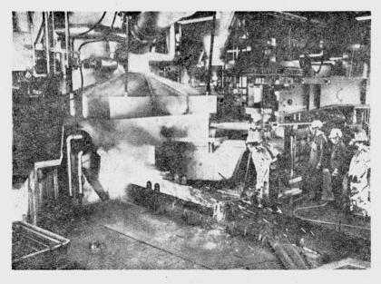
The ScanDust plant is recovering valuable metals such as zinc, lead, chromium, nickel, molybdeum and iron at the rate of 35 000 t/p.a. from the waste oxides in 70 000 t/p.a. of baghouse dust from steel plants throughout northern Europe. Until the PLASMADUST process was developed, the dust was normally piled in waste heaps around the steelworks where it was liable to pollute ground water reserves. The new process is environmentally clean.
