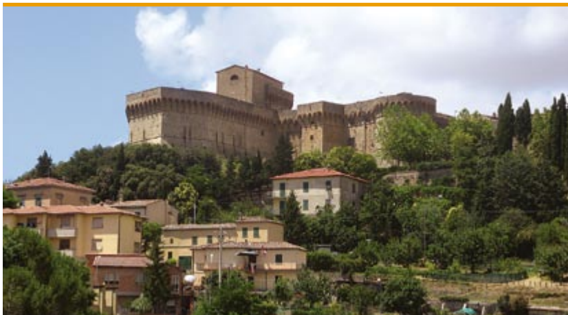
Mury obronne Volterry
