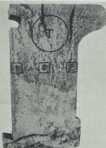
Fig 1 section de rupture
