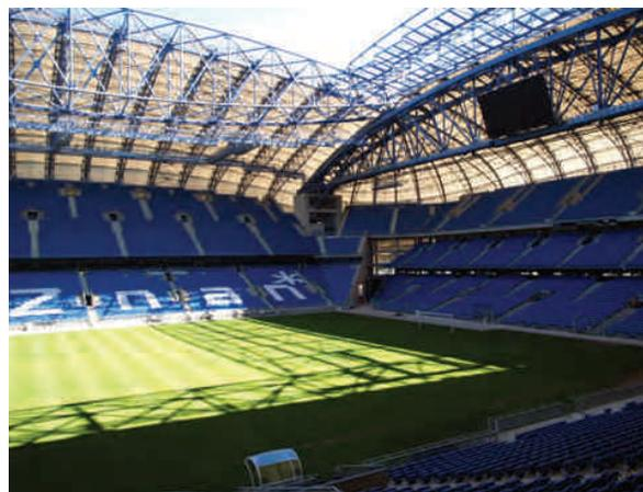
Fig. 3A. Photo of the interior of the stadium in Poznań and the view of the primary 160m long truss with the secondary 135m long, elliptical truss supported on it. The photo shows the “optical ballast” suspended above the heads of thousands of viewers (photo: M. Pelczarski)
