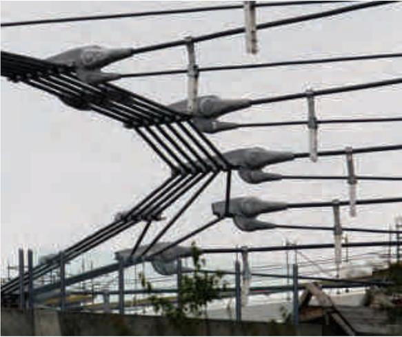
Fig. 9A. View of two clamps which broke while raising the cabling.
