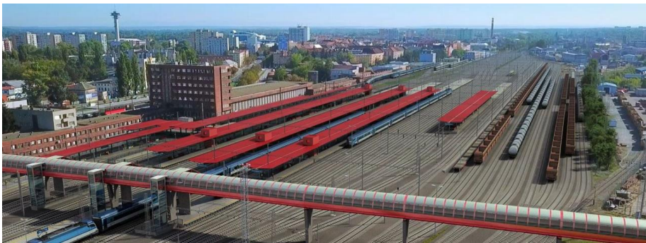
Fig. 3. Pardubice junction after the reconstruction [4]
