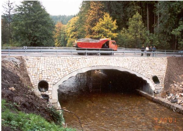
Fig. 4. Side view of bridge and scaffolds for measuring displacements during field load tests during stage 2 (load scheme III)
