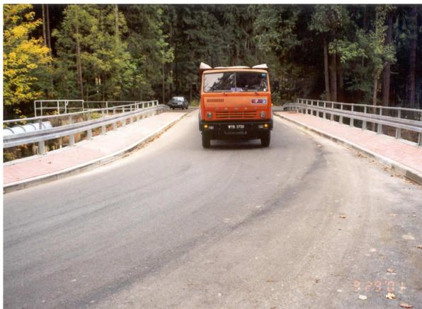
Fig. 3. Front view of bridge during test stage 2 (load scheme II)
