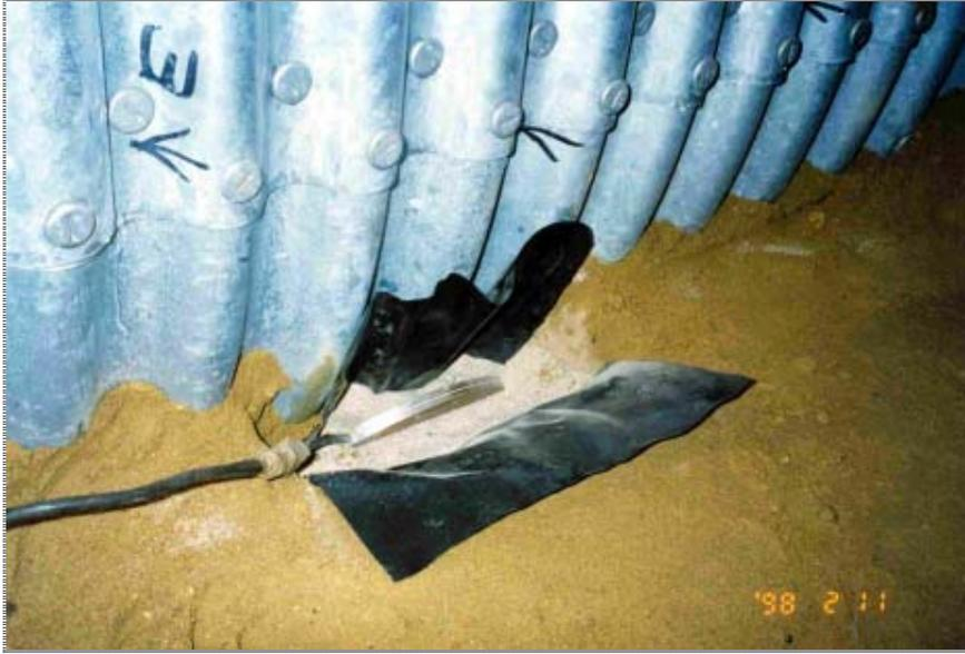
Fig. 6. View of earth pressure cells during installation
