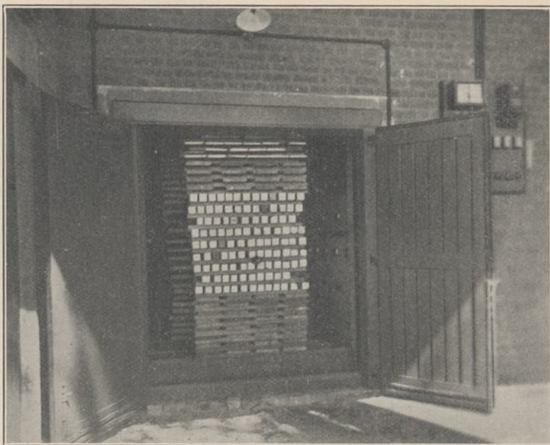
FIG. 2.—Experimental Sturtevant kiln at the Forest Research Institute, Dehra Dun, showing timber stacked ready for seasoning.
