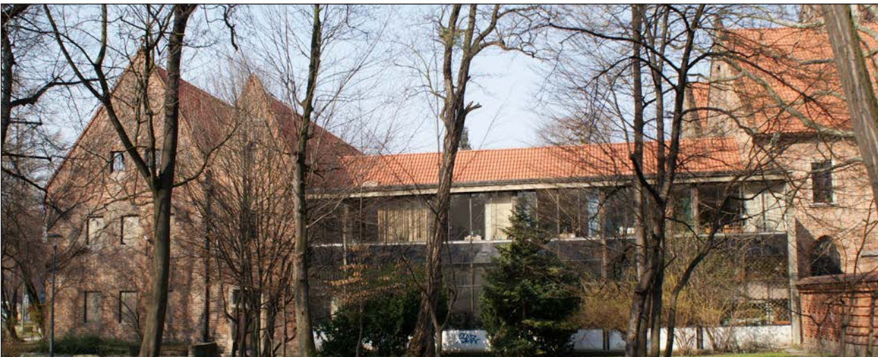
79. East wing of the former post-Bernardine monastery, external façade (2015); photo: E.G.
