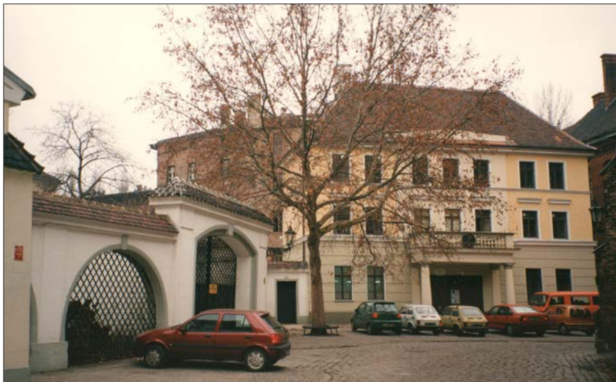
128. View of the southern elevation of the building at 11 Kanonia Street with a fence; from the archives of the Małachowicz family
