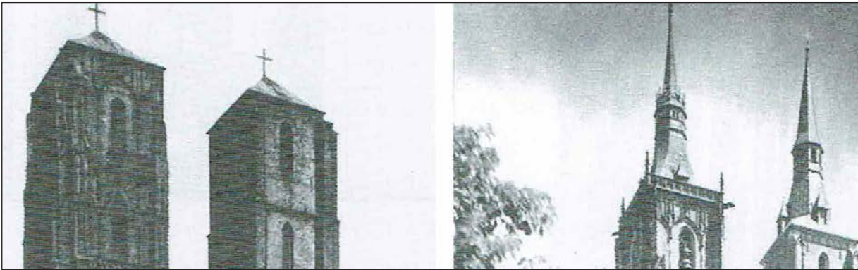
136. Tower spires of Wrocław Cathedral before and after restoration works were carried out (1908–1922) – so-called Hartung’s spires [79, p. 154]
