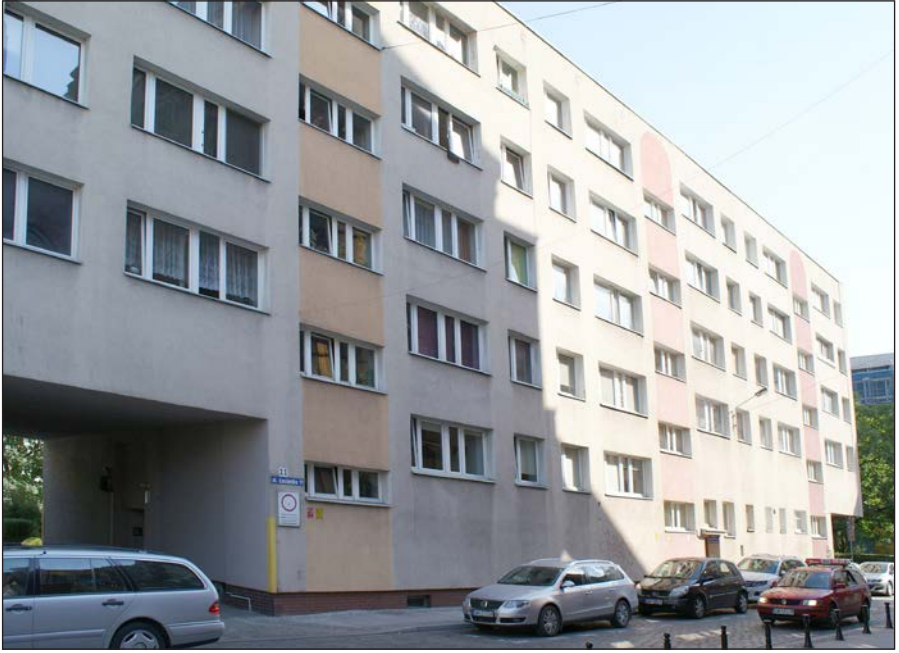
58. Façade from the side of 10-12 Łaciarska Street and a view from the kindergarten side (2018); photo: E.G.
